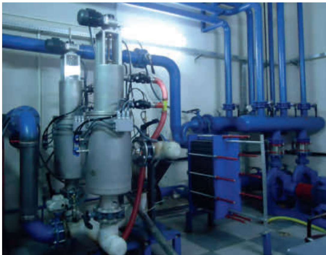
▲ Water Filtration for Protection of Heat Exchanger 90 m 3 /h x 2 nos filters, 500 micron. Photo courtesy of Filternox.
