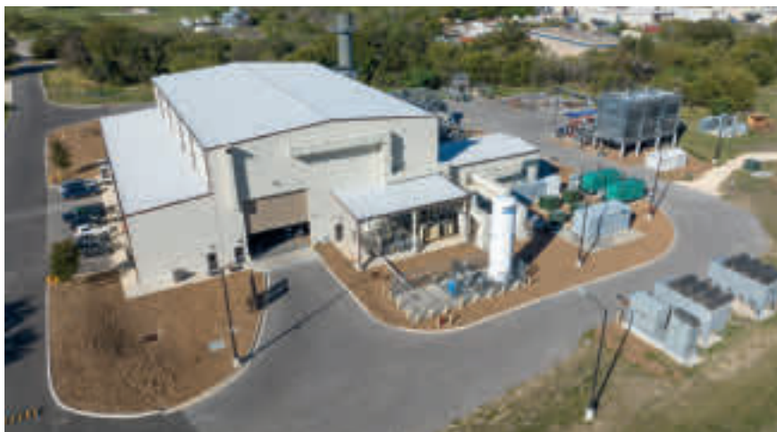
▲ The 10 MWe STEP Demo project in San Antonio, Texas, USA in 2023. In October 2024, the STEP Demo facility accomplished the phase 1 testing milestone: achieving full operational speed of its turbine at 27,000 RPM operating at 500°C. It generated 4 MWe net of grid synchronized power.
