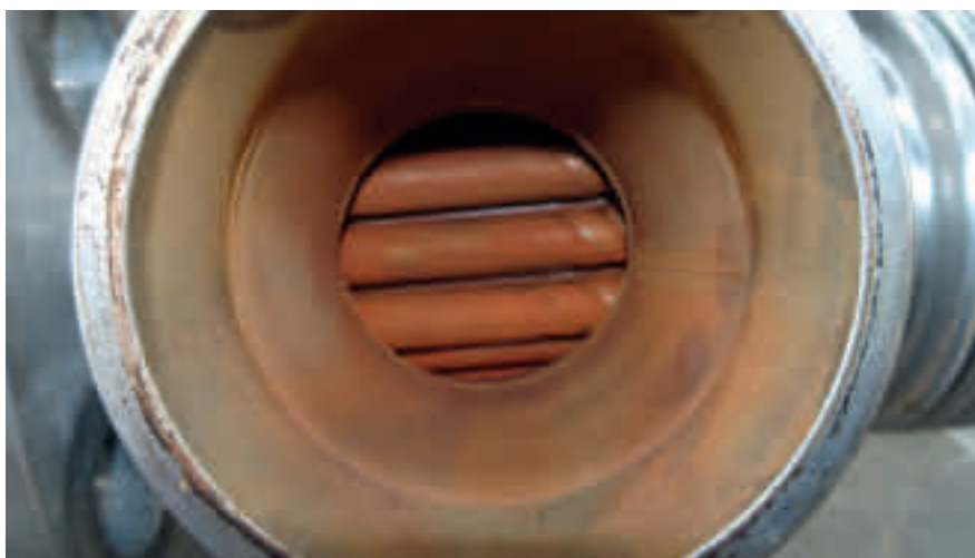
Figure 13. Detail of the service inlet nozzle of a unit with untreated water.
