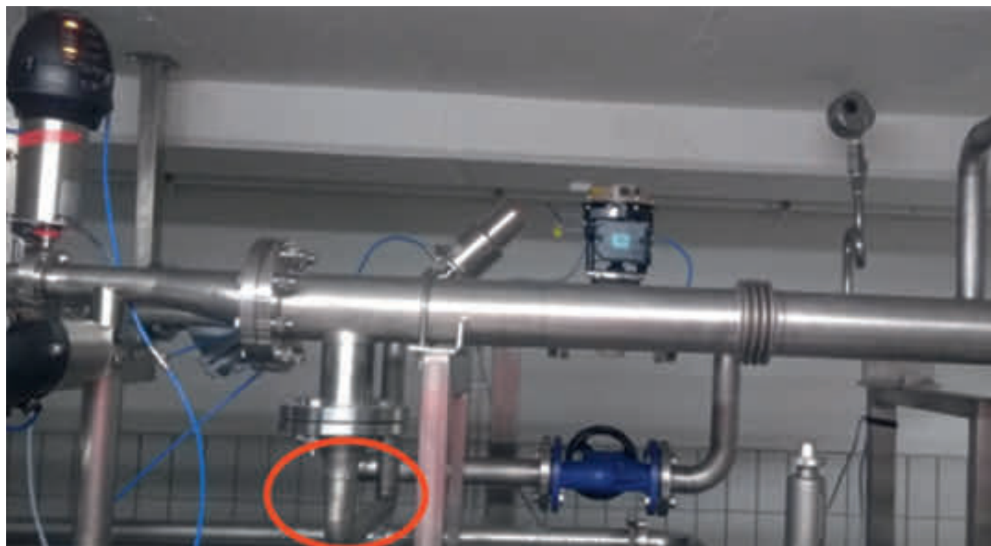
Figure 10. Condensates pipeline with a poor design.
